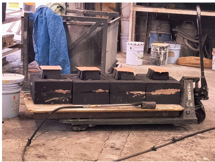
Figure 8. Four molds prepared and positioned for pouring.
