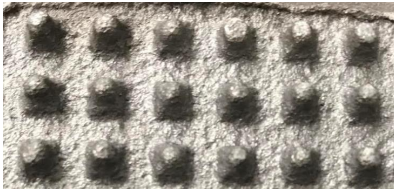
Figure 21. Hammer studs after testing
